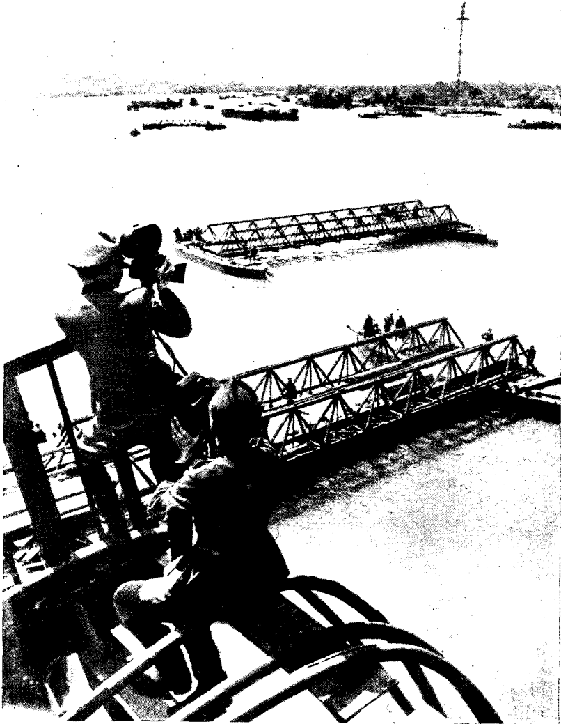
Figure 125.—Photographing Herbert bridge.
